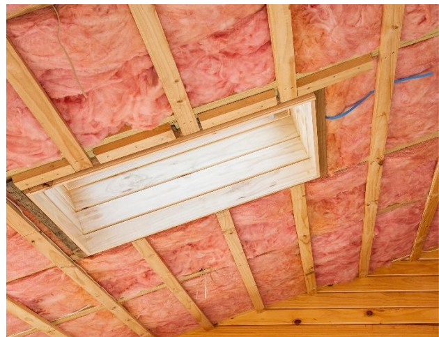
Figure 4. Silica sand, limestone, soda ash, borates, kaolin, lithium minerals, potash, feldspar, fluorspar and sodium sulfate are all used to make fiberglass insulation.
